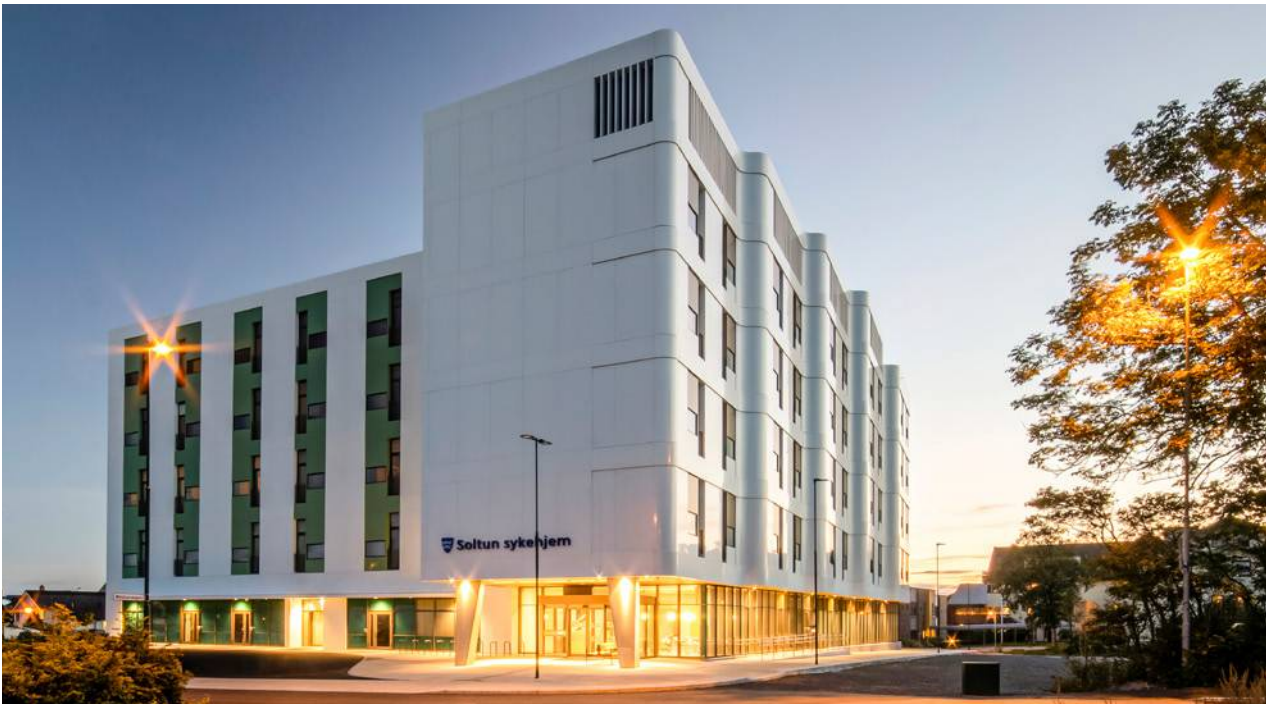
Sola Sykehjem Hospital | Sola, Norway | STB - S10
